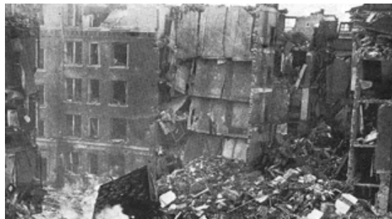
The bombs destroyed many buildings burying mothers, fathers and children in the rubble
