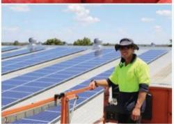
A produce coolstore in Shepparton, Victoria installed a 100kW solar PV roof-mounted system which, along with other energy efficiency upgrade measures that reduced energy use by 25 per cent.
